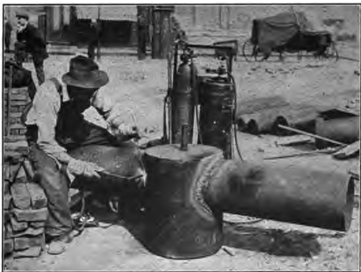
FIG. 76.—Welding with oxy-acetylene blow-pipe. A completed weld shown at the right.
